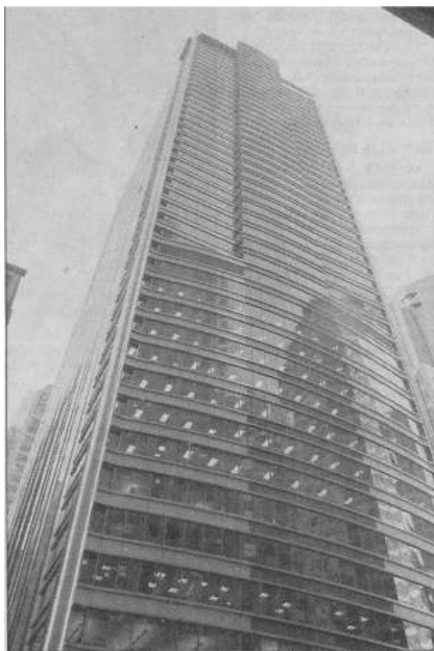
Tribune photo by Charles Osgood The Wacker Drive facade of the new skyscraper features a gently bowing wall of glass that extends out from the lower 16 stories.
